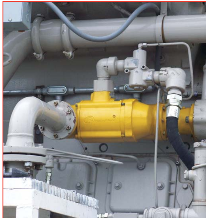
The ST1099CP03R25 is piped for use on a Waukesha 7044 gas compression package.
